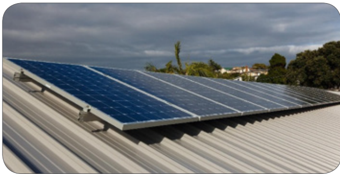
Figure 1: An example of a framed PV panel mounted above a steel roof
