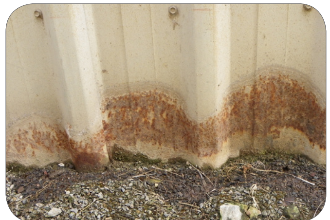
Figure 3: Corrosion due to soil immersion
