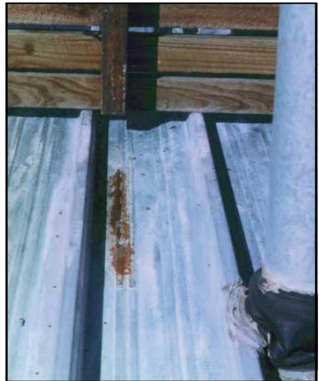
Figure 1: CCA treated timber walkway
