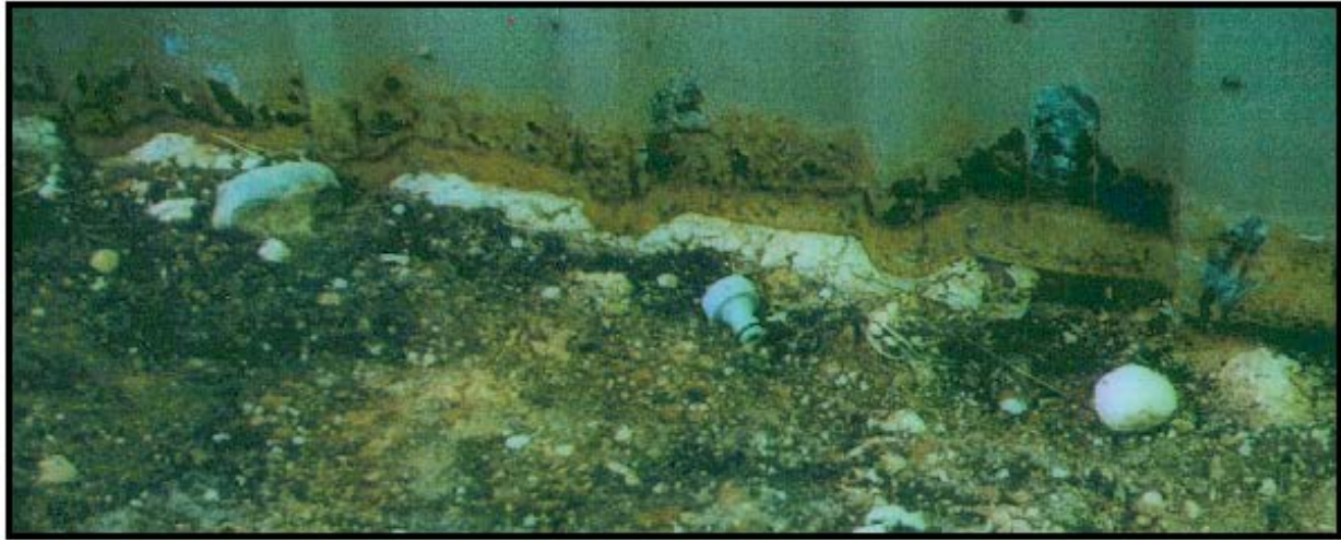
Figure 1: Immersed Shed Wall
