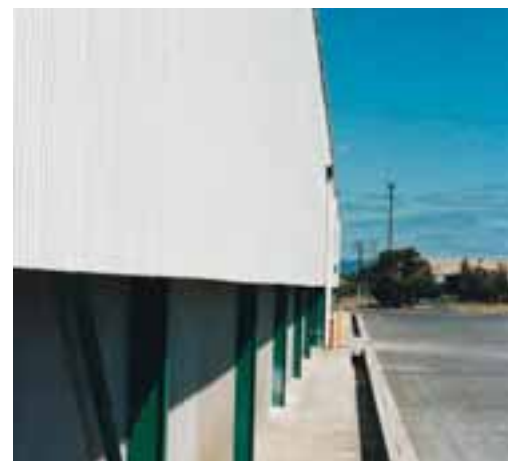
Figure 3: Example of a dwarf wall
